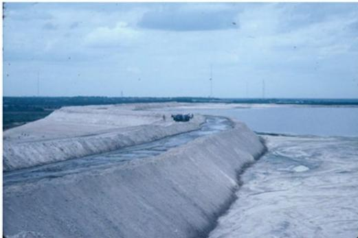
Fig 3 (a) Elevated sloping rim ditch
