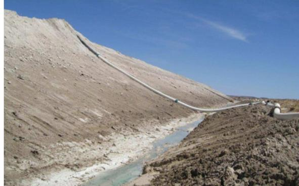
(b) HDPE slurry line to stack top
