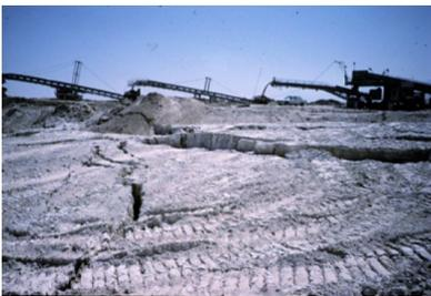
Fig 9 (a) Cracks in dry stack on level ground
