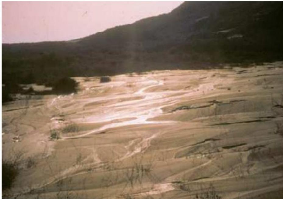
Fig 10. Seepage from the base of a dry stack
