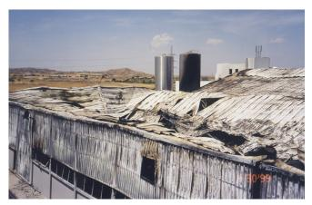
TOTAL LOSS OF A DAIRY PLANT CONSTRUCTED OF PU FOAM INSULATED SANDWICH PANELS
