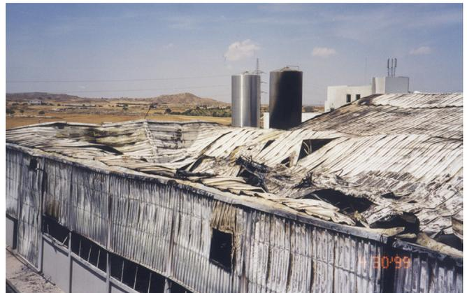
**TOTAL LOSS OF A DAIRY PLANT CONSTRUCTED OF PU FOAM INSULATED SANDWICH PANELS**
