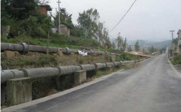
Fig 1 (a) High pressure gypsum slurry pipeline
