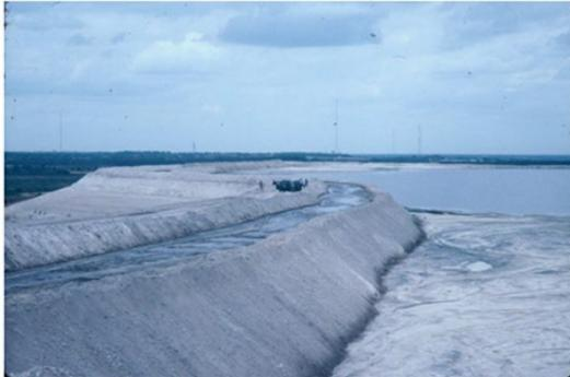
Fig 3 (a) Elevated sloping rim ditch
