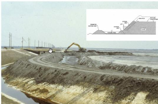
Fig 4 (a) Upstream method of construction
