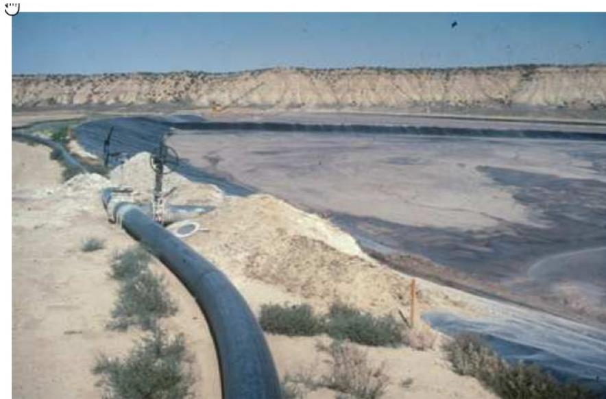
Fig 5. Gypsum slurry deposition using spigots
