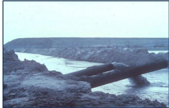
(b) Gypsum slurry discharge to rim ditch
