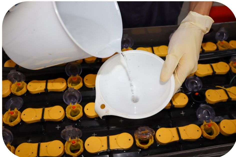
Flooded cell lead battery electrolyte maintenance (replenishing lost water)
