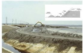
Fig 4 (a) Upstream method of construction
