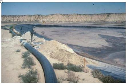
Fig 5. Gypsum slurry deposition using spigots
