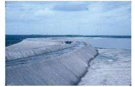
Fig 3 (a) Elevated sloping rim ditch
