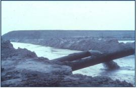
(b) Gypsum slurry discharge to rim ditch
